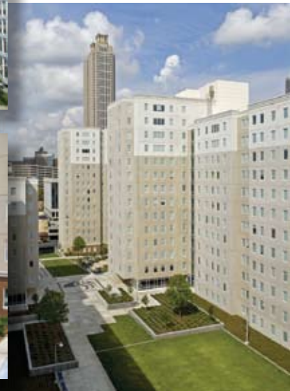
The sheer size of the University Commons project at Georgia State University magnified any design decisions, resulting in the project team selecting non-load-bearing precast concrete sandwich wall panels with 4 in. of expanded polystyrene insulation.
